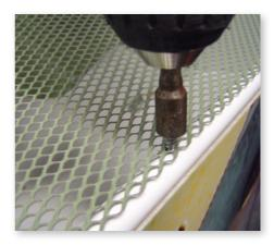
NOTE: Make sure never to over tighten any of the screws. The product only requires positive pressure to secure it in place.
