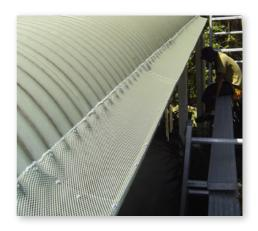
It is important that the product is manufactured with a fold to reduce the angle of the mesh. If the mesh is to steep above the gutter, water will overrun the mesh and not fall through into the gutter.
