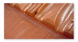
Terracotta tile. Nose of second row tile to flat product, sealed edge. Important to make sure the mesh hole openings face away from the roof for debris to slide over the gutter edge.
