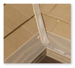
Flat tile, internal corner, with valley, cut & sealed.
