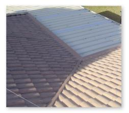
Close up of a sealed concrete tile valley. Leaves a clear path for water to flow to the gutters
