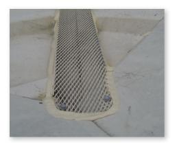
Alternate, over the top method. Cut & seal.
