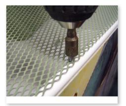
NOTE: Make sure never to over tighten any of the screws. The product only requires positive pressure to secure it in place.
