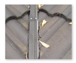
NOTE: It may be necessary to hand bend the product to aid in the installation if the gutter lip is lower in reference to the roof line. (See Tips Section)
