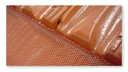
Terracotta tile. Nose of second row tile to flat product, sealed edge. Important to make sure the mesh hole openings face away from the roof for debris to slide over the gutter edge.
