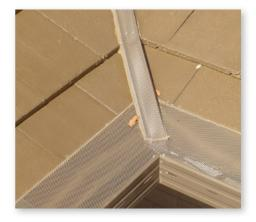
Flat tile, internal corner, with valley, cut & sealed.
