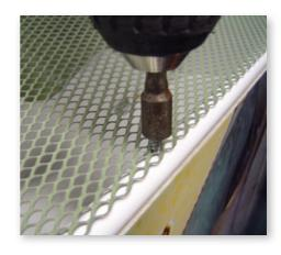
Class 4 Self drilling Fasteners are required as a 'minimum' under the Australian Standard for the building & construction industry.
